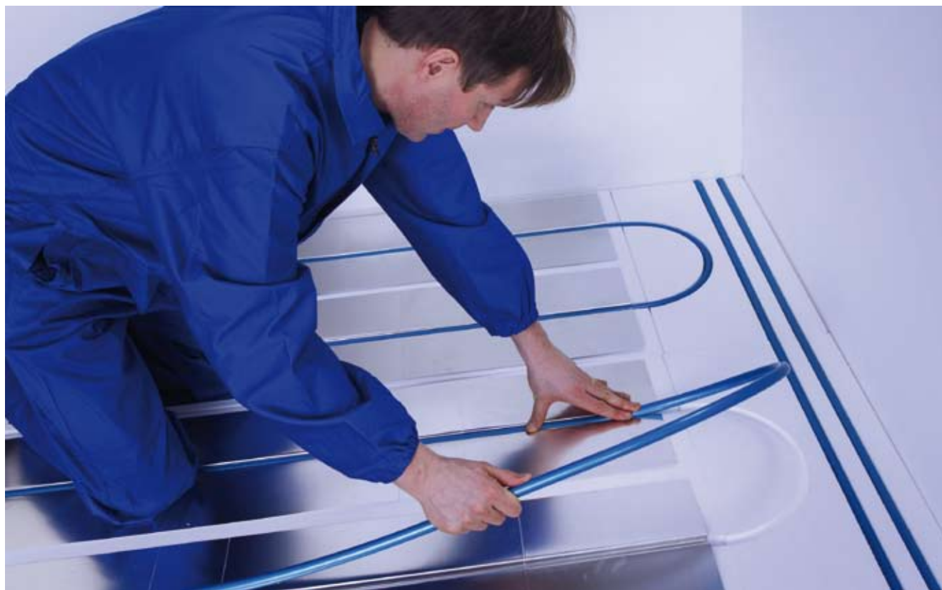
Installation of Thermotech Floating floor
