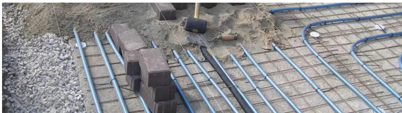
Installation of Thermotech snowmelting system
